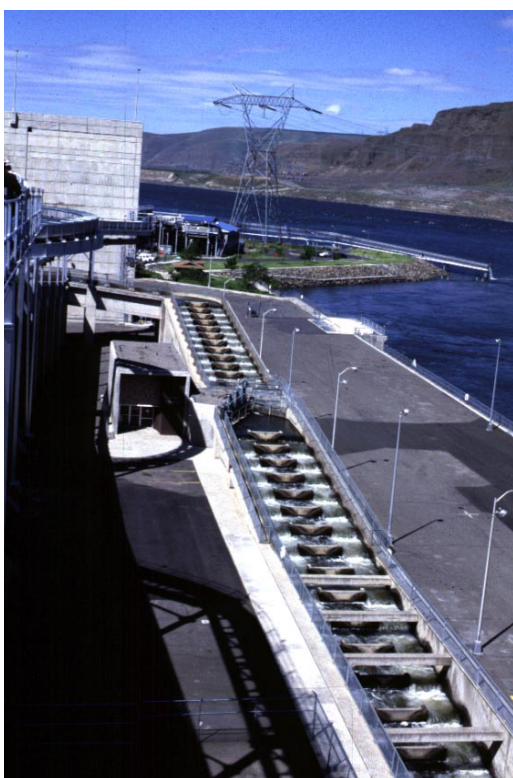
Figure 1. Fish Ladder at Little Goose Dam
